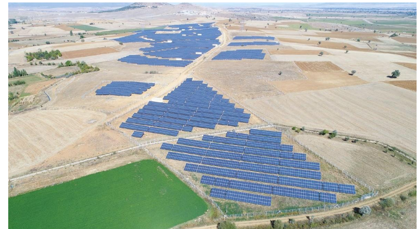
SEYDISEHIR SOLAR POWER PLANT Established DC Power: 13.000,00 kWp
