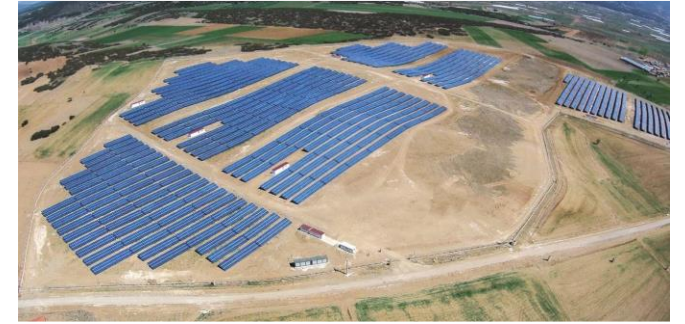
DIANA ENERGY GOLHISAR SOLAR POWER PLANT Established DC Power: 8.800,00 kWp
