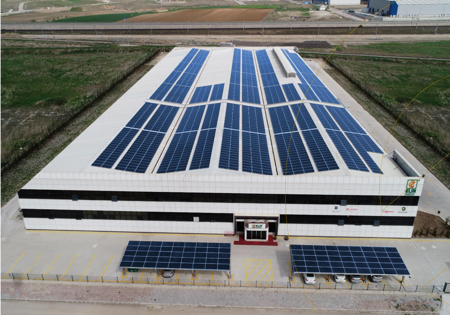
ELIN ENERGY PV MODUL FACTORY IN ANKARA
