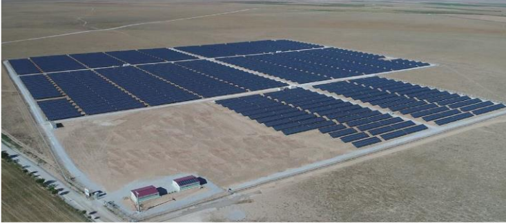
ME-SE SOLAR POWER PLANT Established DC Power: 12.094,83 kWp
