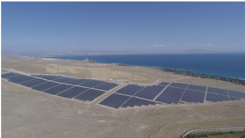
OMICRON SOLAR POWER PLANT Established DC Power: 24.189,66 kWp
