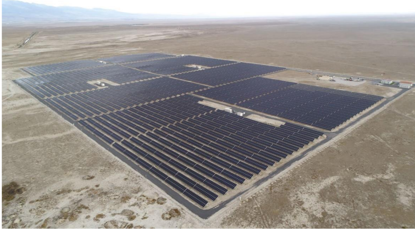
AFTA & SOLANA SOLAR POWER PLANT Established DC Power: 17.253,00 kWp
